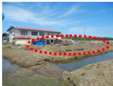
Project Site (Before)
