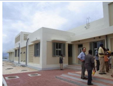
Fish Handling Building (Aug, 2011)
