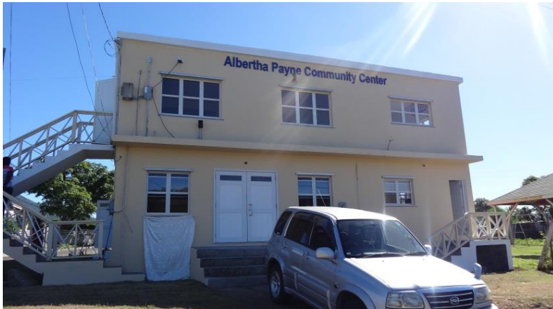
Newly renovated Albertha Payne Community Centre
