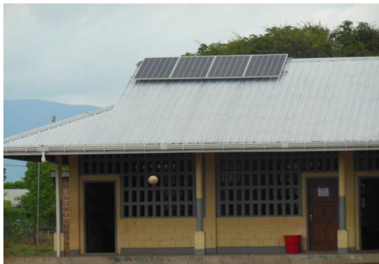
The St. Ignatius Secondary School, beneficiary of solar panel systems funded by the Embassy of Japan GGP scheme.
