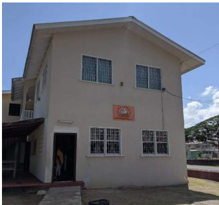
VYC Youth Center, which will be renovated under the project
