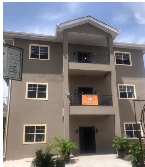
Photo of VYC Youth Center after renovation
