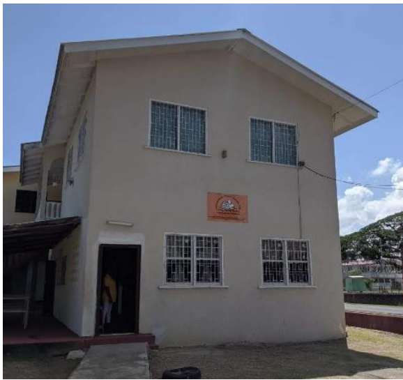
Photo of VYC Youth Center prior to renovation
