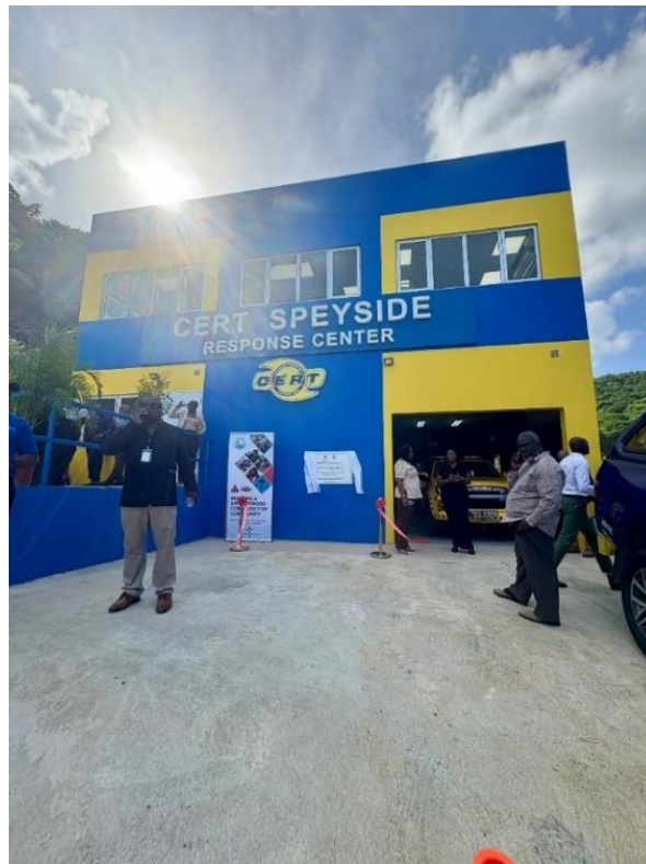
Newly constructed CERT Speyside Response Centre.
